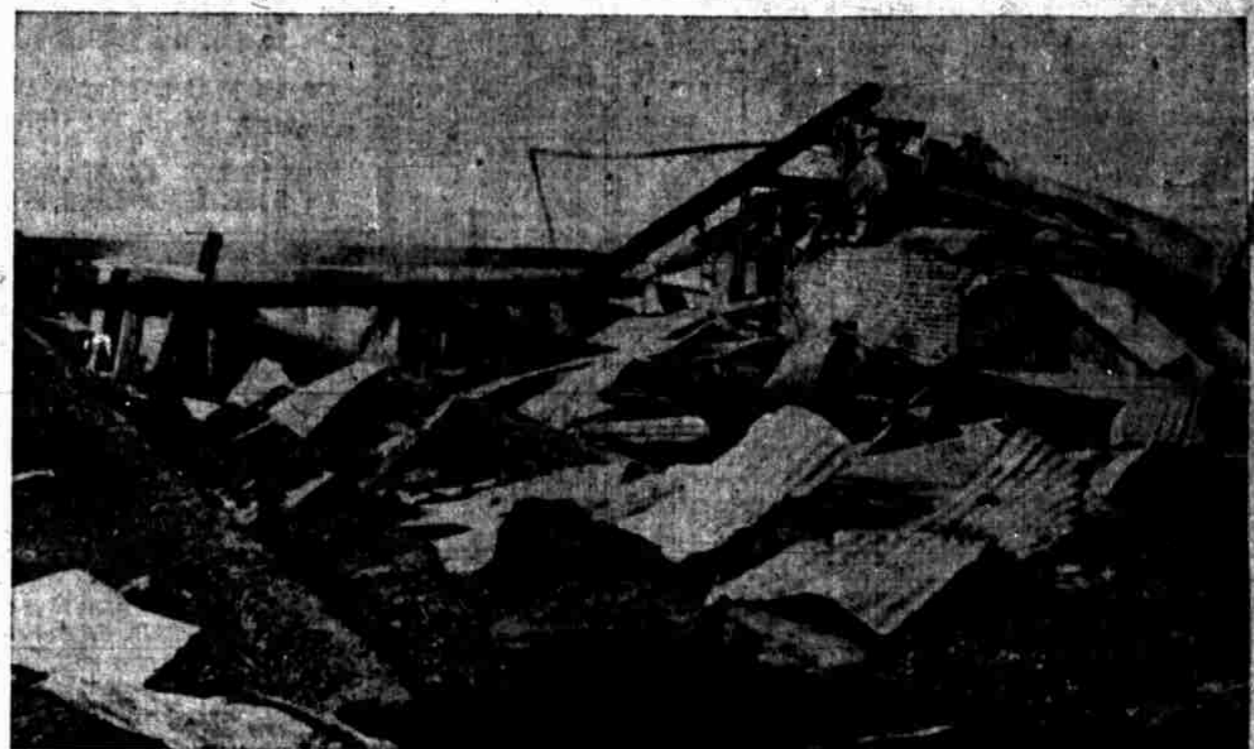
St. Johns Lumber Mill, After the Fire
