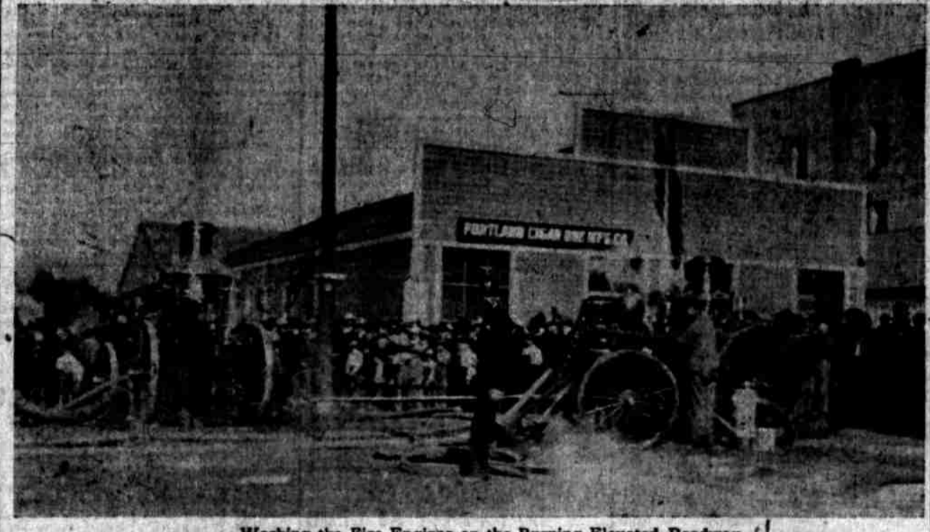
Working the Fire Engines on the Burning Elevated Roadway.
