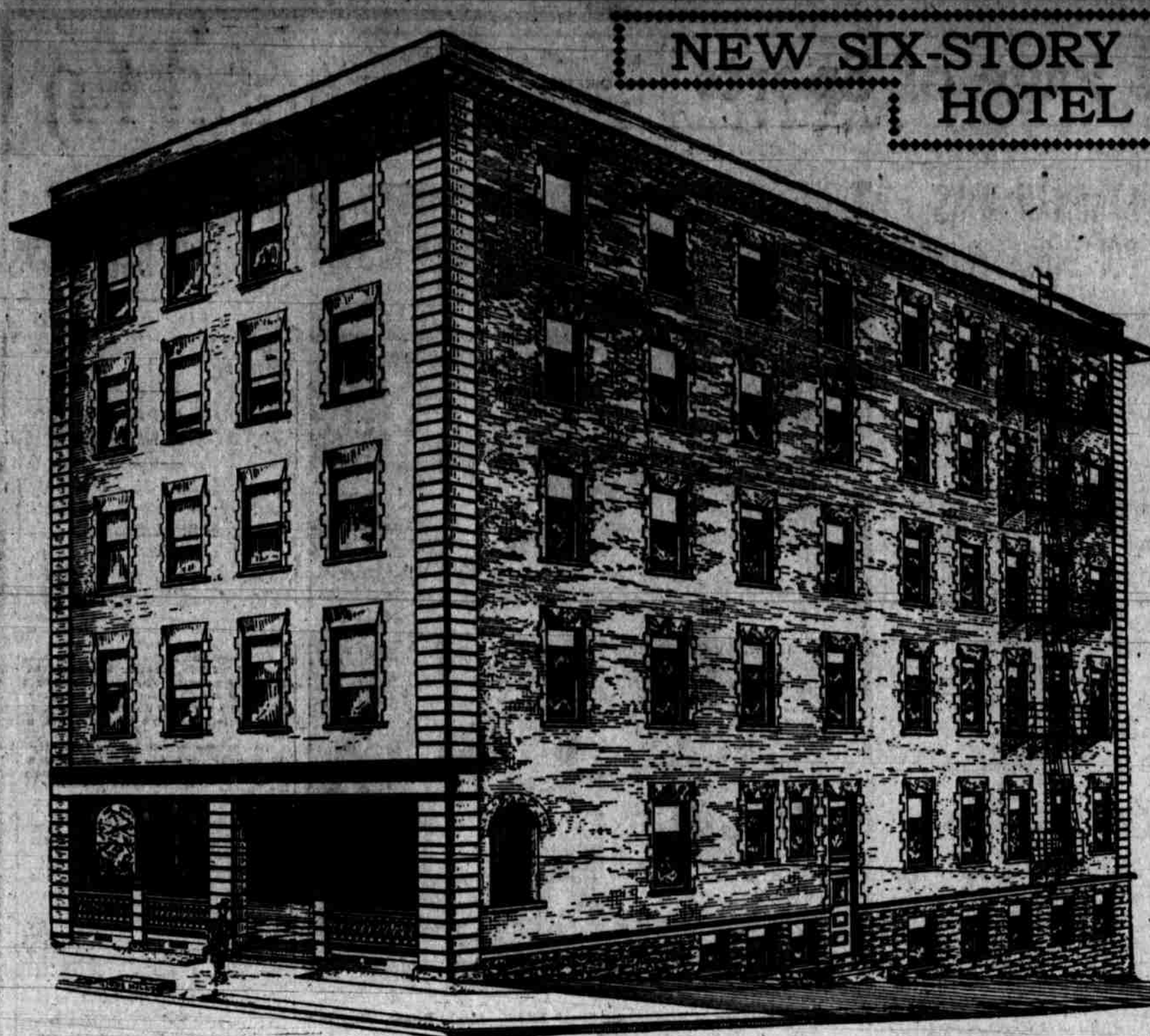
Hotel Being Built by S. Silverfield.
