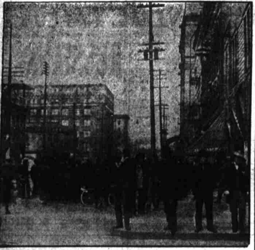
AN EXAMPLE OF THE WAY IN WHICH STREET FAKERS BLOCK THE STREETS. (Photo by Kiser Bros.)
