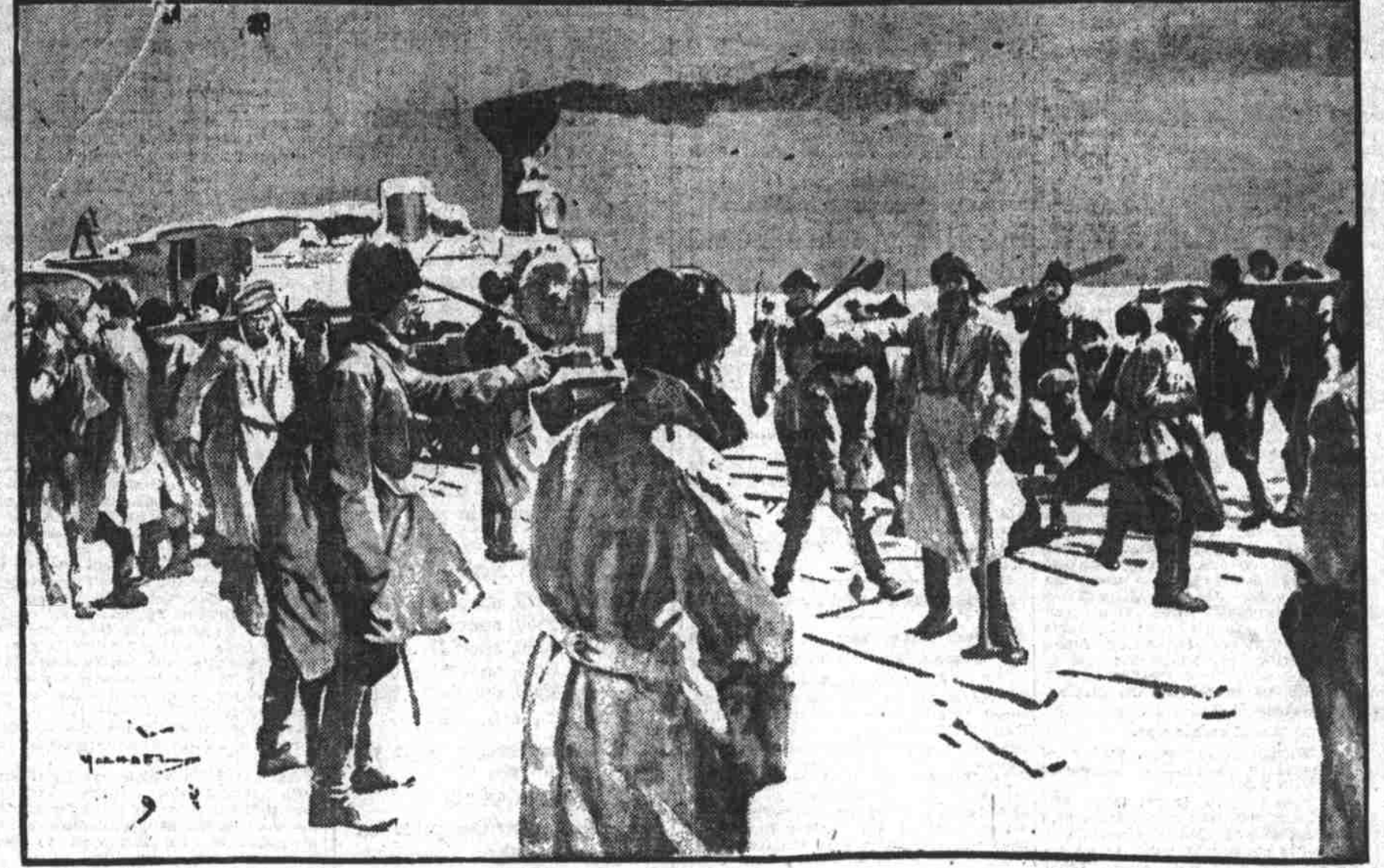
This picture, from a photograph recently received here, shows the Russians building a railroad across the ice on Lake Baikal. This gap in the trans-Siberian road has given the Russian authorities much worry.
