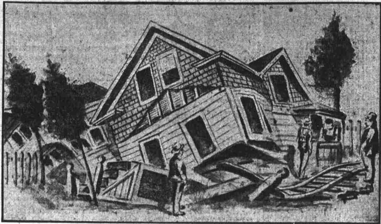
T. W. STARBUCK'S HOME WRECKED BY THE STORM.
