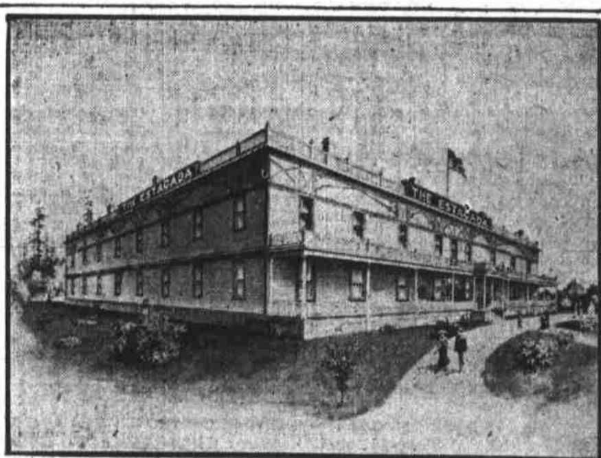
ESTACADA HOTEL, NOW NEARING COMPLETION.
