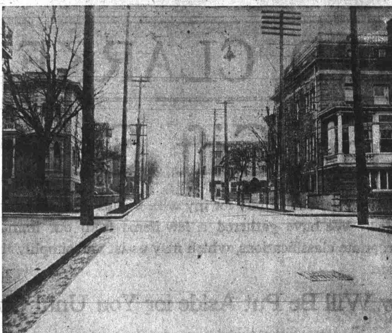
ASPHALT PAVEMENT. ALDER STREET, LOOKING WEST FROM PARK STREET.
