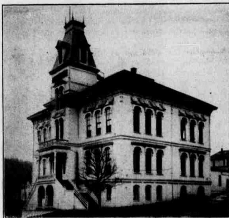
ASTORIA HIGH SCHOOL BUILDING.
