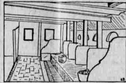
Cow Stable in Scotland—Double Stalls Are Divided by Glazed Tile Partitions—The Floor is Paved With Brick and is Scrubbed Daily.
