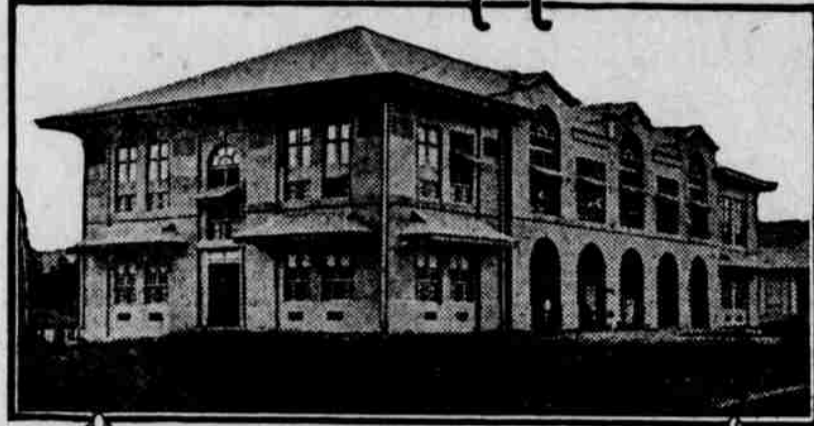
HIGH SCHOOL BUILDING, CEBU
