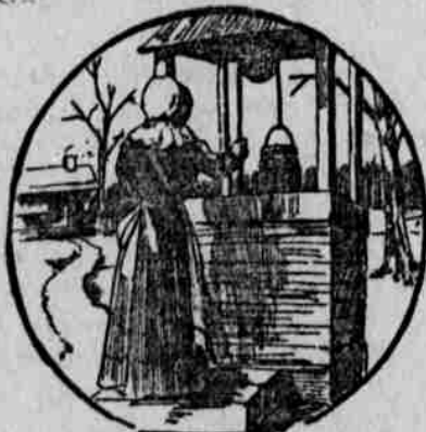
Antiquated Water System.
