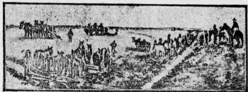
SCRAPERS AT WORK ON GOVERNMENT IRRIGATION CANAL.
