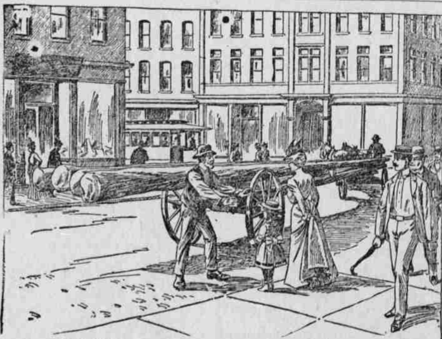
PILOTING LONG POLES THROUGH THE STREETS.
