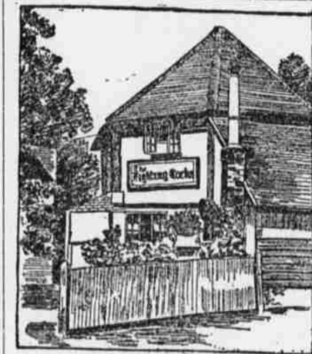
REBUILT AFTER THE FLOOD.
