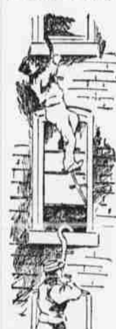
FOUR-MEN LADDER DRILL.
