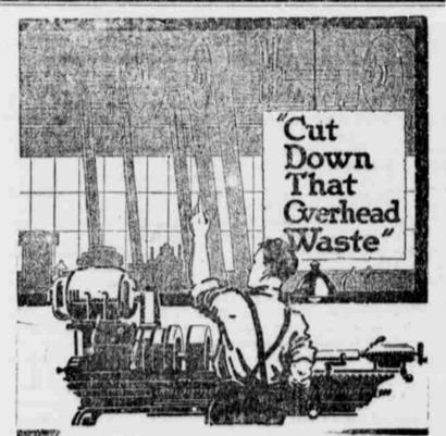
ELECTRIC DRIVE ELIMINATES LONG LINES OF OVERHEAD SHAFTING, which represents a dead loss in efficiency of as much as 6 per cent.
