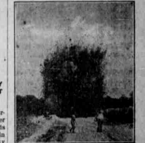
THE BLAST THOROUGHLY CRACKS THE SOIL, BUT USUALLY LEAVES A CAVITY OR POTHOLE AT THE BOTTOM—THIS MUST BE FILLED.
