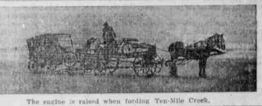
The engine is raised when fording Ten-Mile Creek.
