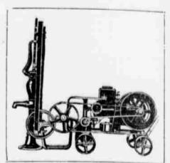
The GILSON 60-Speed Gasoline Engine, made in 1 3-4 and 3 Horsepower, mounted on hand truck as shown, complete with line shaft, pulleys, pump jack and belting. By changing pulleys 60 different speeds, ranging from 167 to 1,500 revolutions per minute can be attained.
