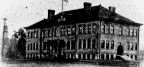
NORTH BEND HIGH SCHOOL.
