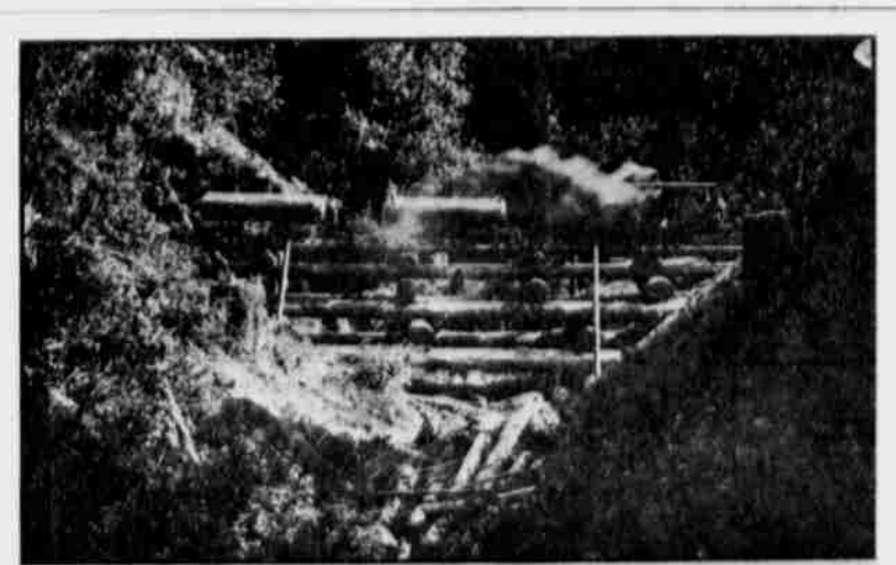
BRIDGE ON LOGGING RAILWAY.
