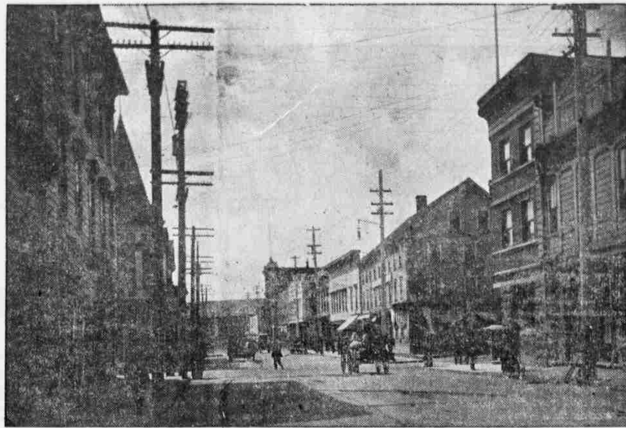
FRONT STREET, SHOWING NEW ASPHALT PAVEMENT AND OTHER IMPROVEMENTS.
