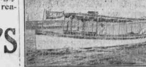
feet six Inches Twenty inches draf Oak frames, planked with three-quarter fir. Oak decks and cabin. Two steering wheels, six Edison batteries, magneto, bilge pump, air tank and whistle, anchor, ropes, lights, cushions in fact, everything. 18 Horse-Power 4-Cylinder 4-
