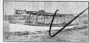
Twenty inches draft. Oak frames, planked with three-quarter fir. Oak decks and cabin. Two steering wheels, six Edison batteries, magneto, bilge pump, air tank and whistle, anchor, ropes, lights, cushions—in fact, everything. 15 Horse-Power 4-Cylinder 4-
