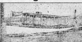
Twenty inches draft. Oak frames, planked with three-quarter fir. Oak decks and cabin. Two steering wheels, six Edison batteries, magneto, bilge pump, air tank and whistle, anchor, ropes, lights, cushions-in fact, everything. 15 Horse-Power 4-Cylinder 4-
