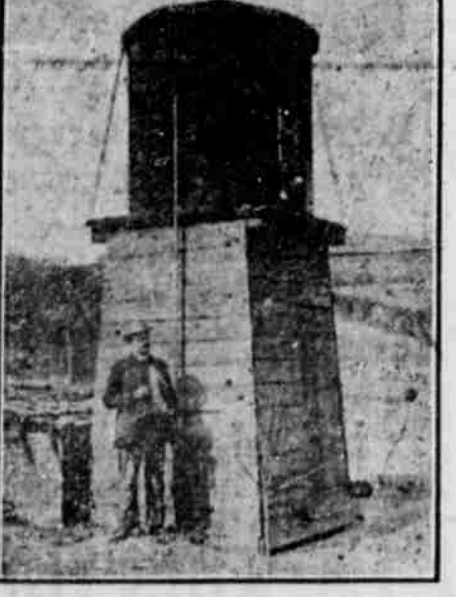
Photo by C. M. Barnitz. OUTSIDE TANK.
