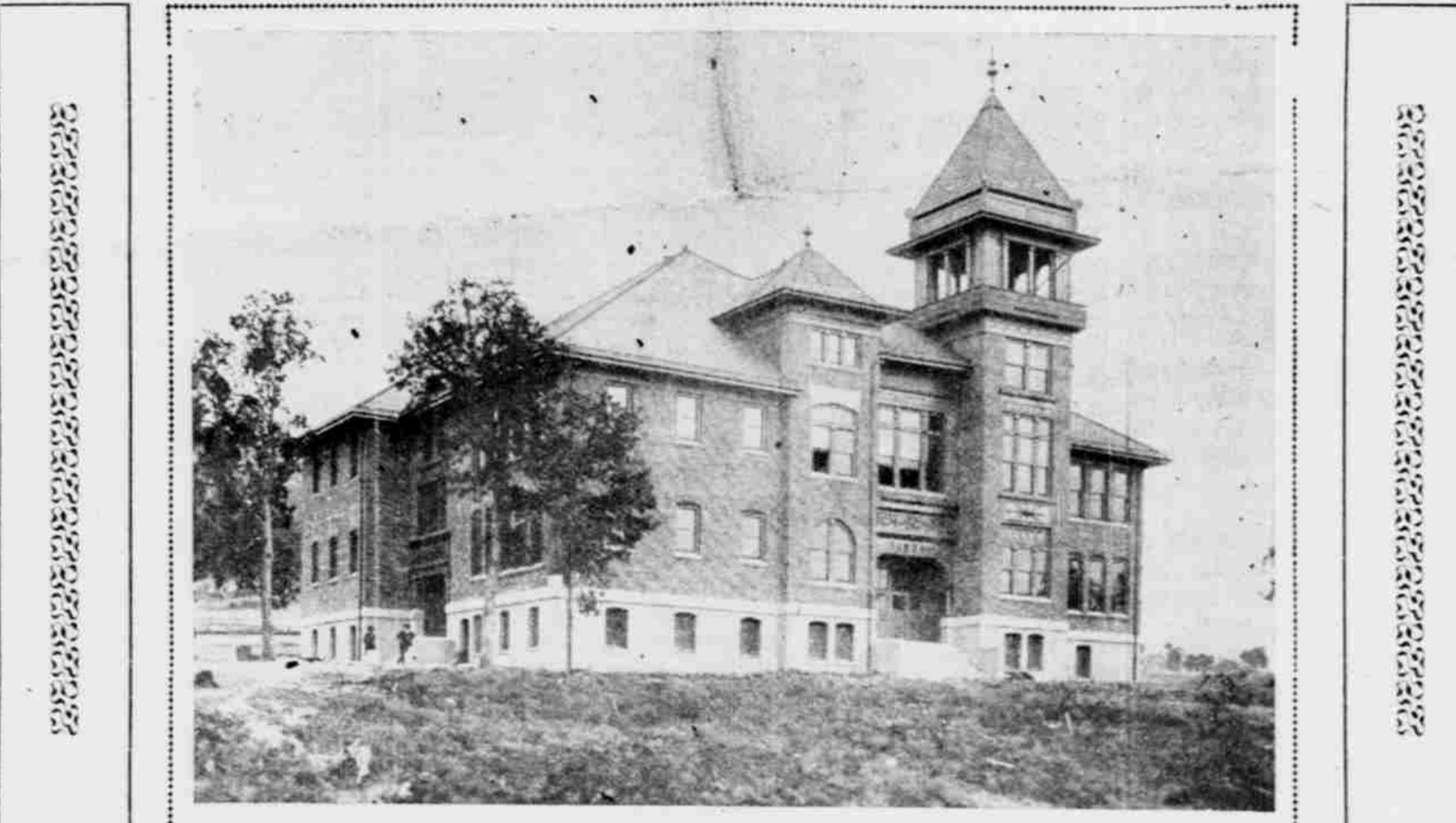
Roseburg's handsome new $25,000 brick High School building is now completed, furnished and ready for occupancy. The building is of brick and modern in every particular, well lighted, heated and ventilated. There are three large entrances to the building, rendering it very easy to escape in case of fire.
