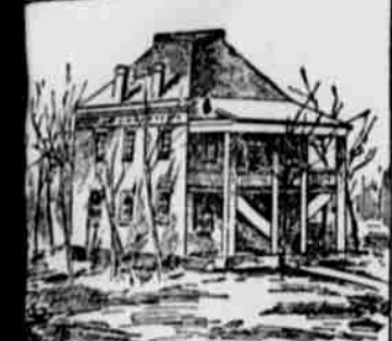
ST. CLAIR COUNTY COURTHOUSE.
