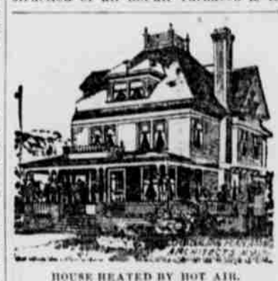
HOUSE HEATED BY HOT AIR.
