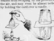
Place two tumblers mouth to mouth, fitting each other, and separate them only by a piece of datep paper. Put a lighted piece of caudle in the lower When it goes out you will see tumbler. When it goes out you will see that the tumblers can be both lifted by the upper one, for the taper has used up nds the tumblers together.
