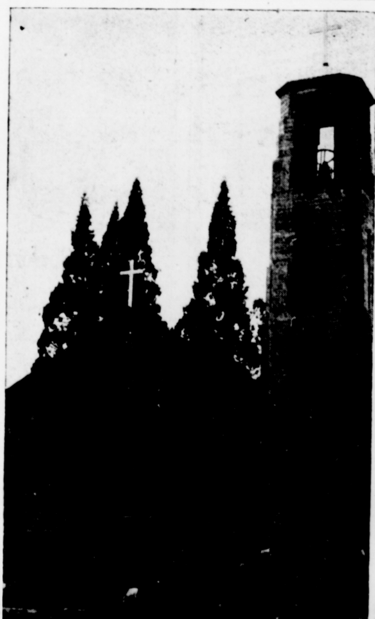
THIS NEW VERBOORT VISITATION church will be dedicated Sunday with appropriate pomp and solemnity. Under construction for 10 months, the church is of concrete and steel construction. Brick veneer will be added later.—(Argus photo by Ernie Martz)
