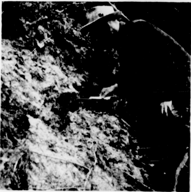
A CRACK IN THE EARTH, resulting from the earthquake, is inspected by County Roadmaster Ross Hartman. The crack, approximately 60 feet long and nearly 10 to 12 inches wide in places, opened on the banks of Dairy creek at the Sussauer bridge, north of Cornelius. Construction was about to begin on a new bridge, but the crack called for a change in plans and caused a need for piling to be sunk in a different location.—(Argus photo by Walt McKinney)
