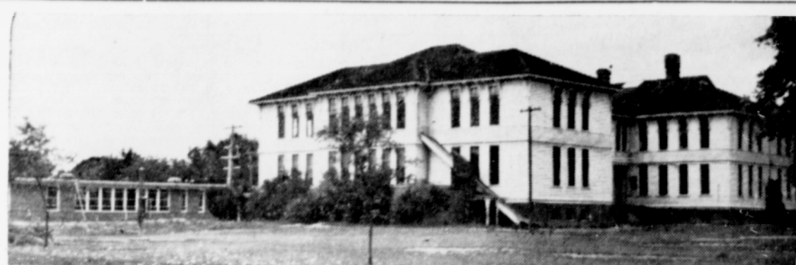
SCHOOL WRECKING SLATED—Bids will be opened August 9 for the wrecking of the old David Hill grade school building, which has served local elementary school needs since before the turn of the century. The venerable structure is pictured above from the Walnut street side. Replacing it is the modern one-story building partially visible at the left.—(Argus photo)
