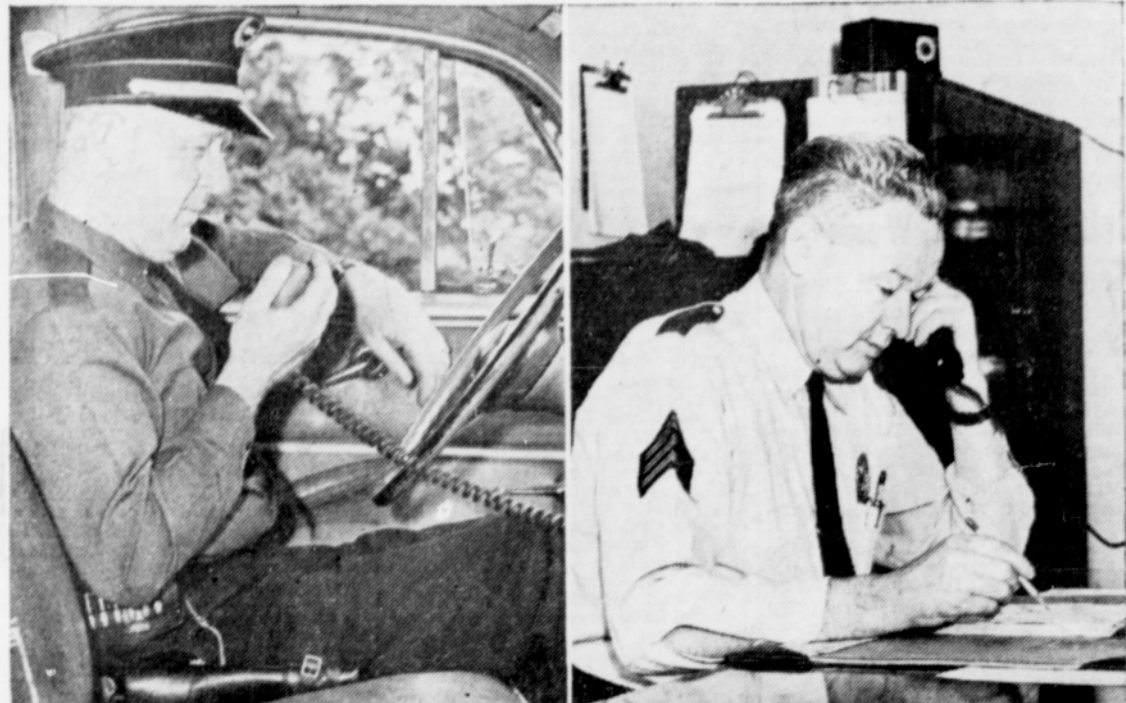
CITY INSTALLS RADIO SYSTEM—Station KGVG, a 250-watt radio station, was installed at police headquarters in Hillsboro recently. Police Chief Melvin DeRock talks over the remote control set from his patrol car to Sergeant George McPherson.—(Argus photo)
