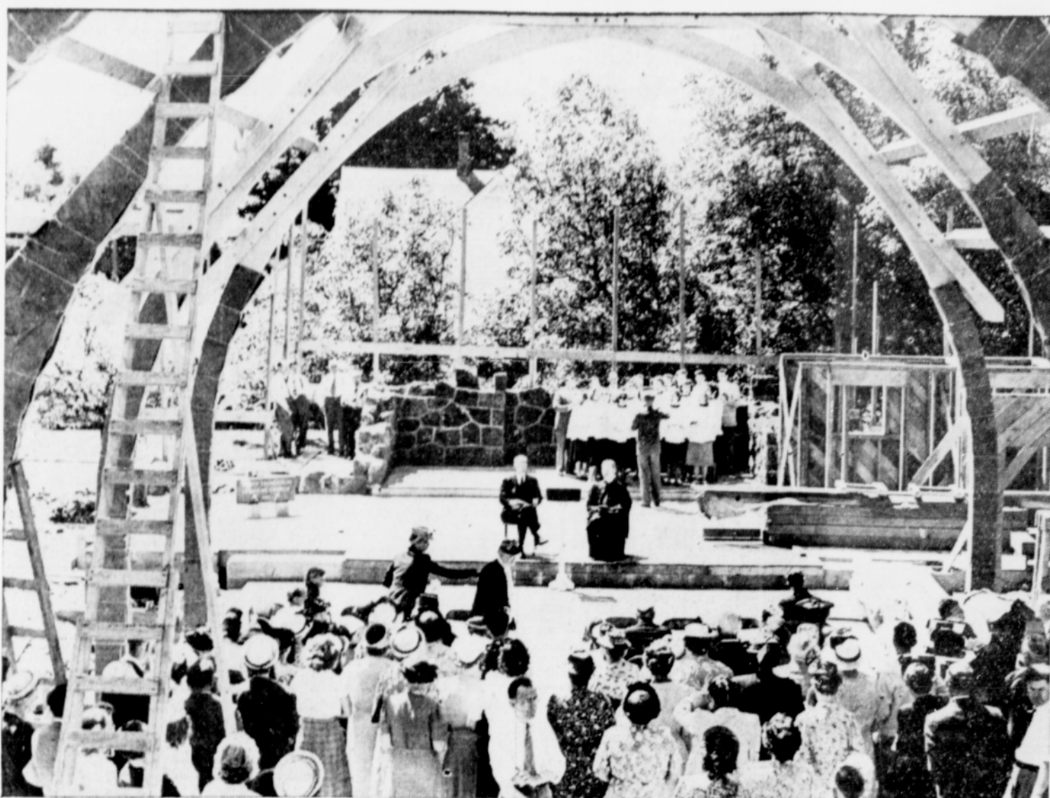
LAYING OF CORNERSTONE—Trinity Evangelical Lutheran church of Hillsboro, located at Fourth and East Main, held cornerstone laying service, Sunday at 3 p. m. The choir, under the direction of Ed Kie-
