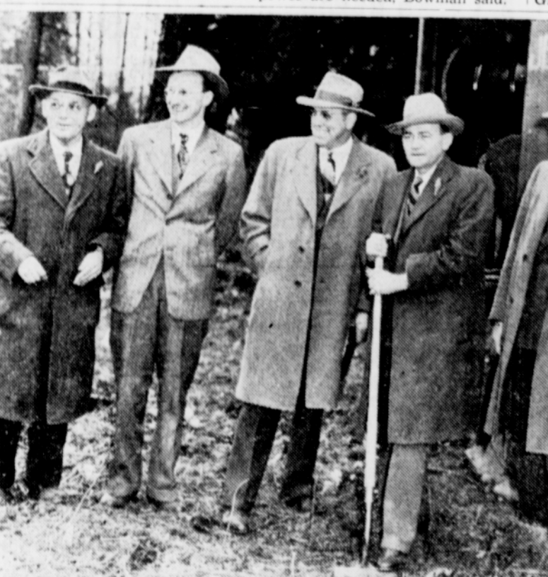
GOVERNOR BREAKS GROUND—Washington county last week was named as the site for one of over 100 Blanding's Dream Houses to be built this spring in every metropolitan area in the nation. Governor John H. Hall is shown above breaking the first ground at the site one mile north of Beaverton. Among officials taking part in the ceremonies were County Judge H. D. Kerkman (second from right), and Commissioner William A. Bowers (right) of Portland. County Commissioners James Lewis and Henry Johnson were introduced. The project is being undertaken by the Portland Home Builders' association in co-operation with the National Association of Home Builders. Completion is expected in July.—(Argus photo)
