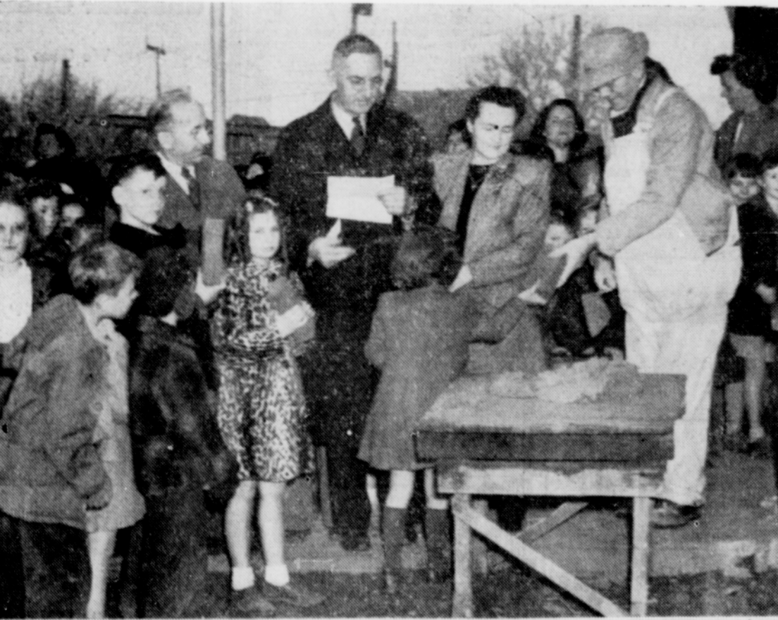
SCHOOL CHILDREN ASSEMBLE FOR CORNERSTONE CEREMONY—David Hill grade school of Hillsboro recessed last week for the laying of the cornerstone of their new school addition. Pupils, representing each grade, contributed bricks to seal up the records that were enclosed in a glass jar and placed in a box. Present for the occasion were (left to right): J. W. Poynter, superintendent of local grade schools; Lester Mooberry, principal; Mrs. Edrie Melhuish, teacher, and Charles Mills of Portland, bricklayer.
