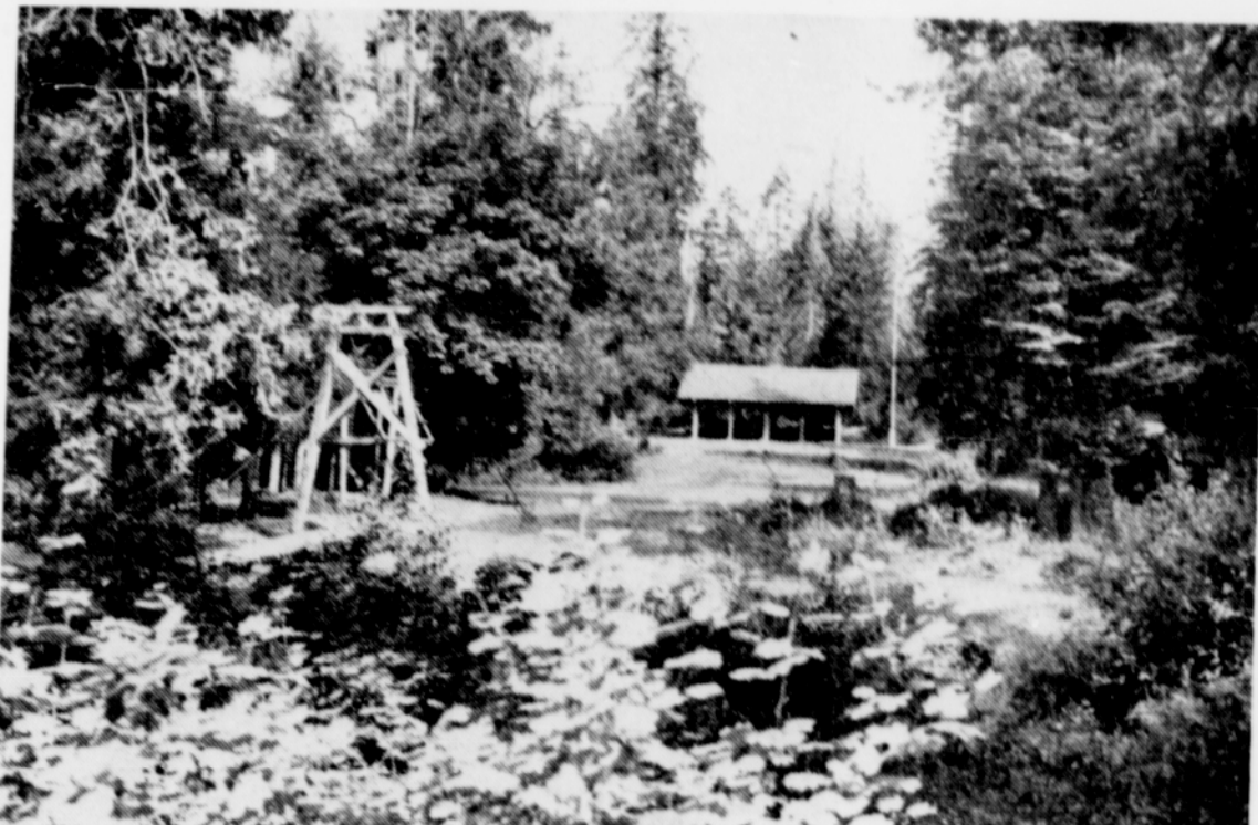
SCOUTS' SUMMER HOME —The big Hillsboro District Boy Scout barbecue to be held next Wednesday evening at Shute park will provide some of the fun as necessary to inaugurate a beautification program for the Boy Scout camping site, Camp Ireland. Located just a few miles north of Hillsboro, the camp needs more parking space, an improved swimming place, enclosure of the pop-wow shelter (shown in background), improvement of toilet facilities, a caretaker's house, a fence around the camp and repairs on the wooden, cable bridge (shown at left).
