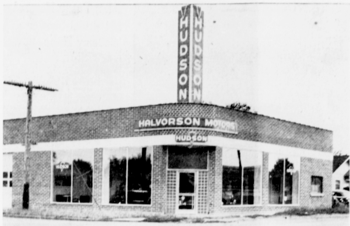
NEW BUILDING COMPLETED —The last accessories to the new quarters of Halvorson Motors were completed Saturday to mark the final completion of this $30,000 building on Baseline and Dennis. Owned by O. C. Halvorson, the 50 by 100-foot concrete and steel building features fluorescent lighting, radiant heat and exhaust ventilation. Construction started in May, 1946, and the Hudson automobile dealer for the county moved in March 1, 1947.
