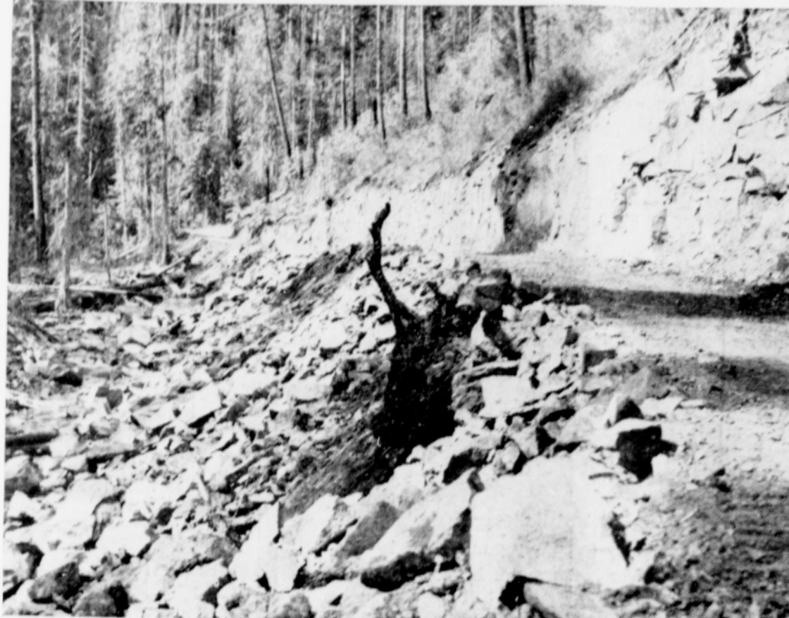
SOLID ROCK DELAYS CONSTRUCTION—Laying of the 18-inch steel pipe along the Tualatin river below Lee Falls encountered such obstacles as solid rock terrain and sectional landlides of loose earth that temporarily prevented progress of trench excavation. Once the cut is accomplished the rock forms an excellent road bed for the heavy type machinery that will travel the road.
