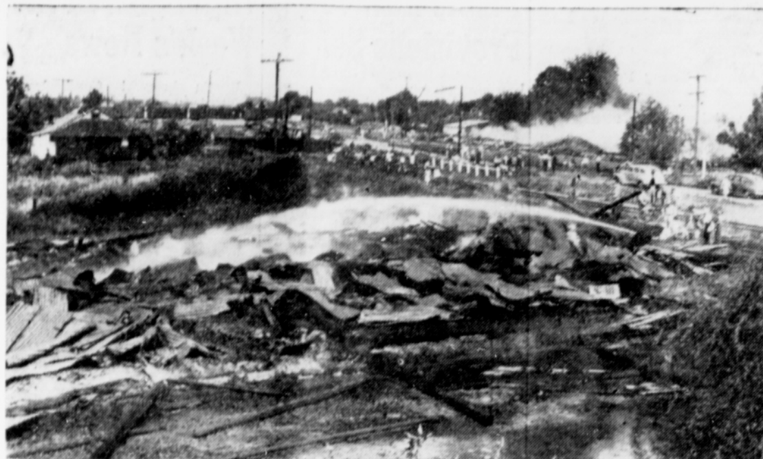
FOLLOWING MORNING'S DEBRIS —All that remained Thursday morning was a mass of smoldering wreckage and grain. Looking west, warehouses were in foreground, SP depot and elevator in the background across the tracks.
