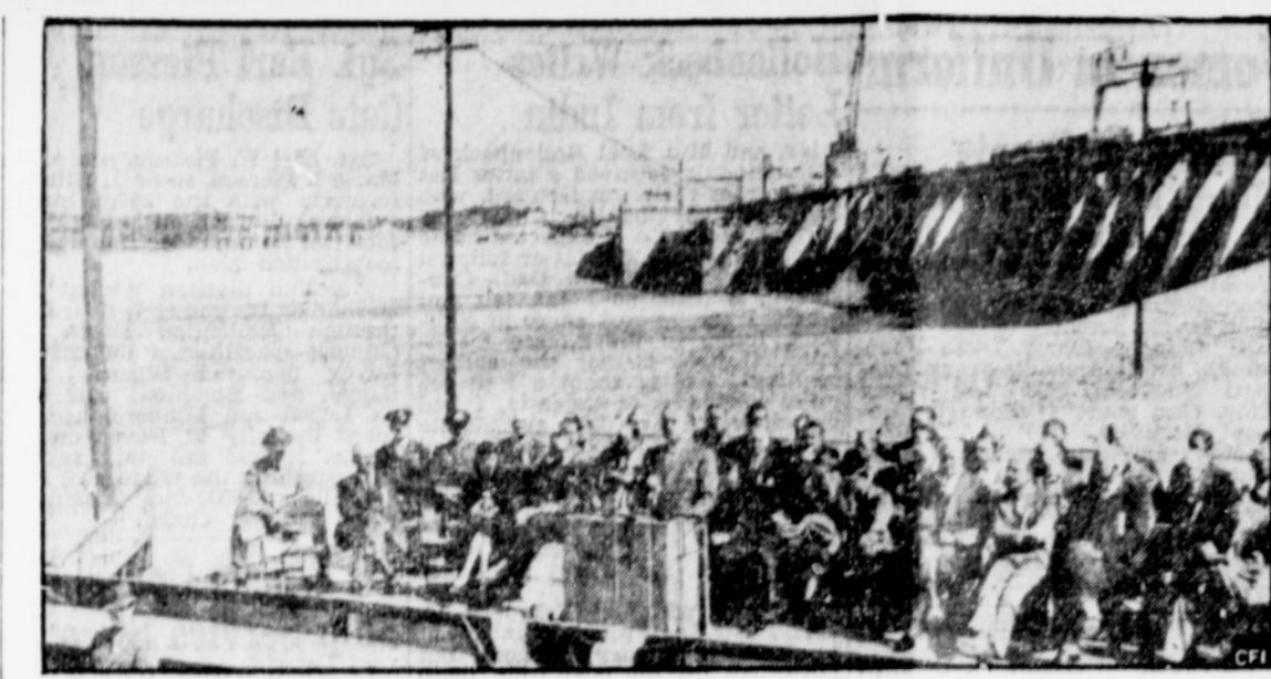
PRESIDENT TRUMAN SPEAKS AT DEDICATION OF DAM—GILBERTSVILLE, Ky.—General view as President Truman spoke at the dedication of the Kentucky dam, last to be completed of the Tennessee Valley Authority project.—(Soundphoto)
