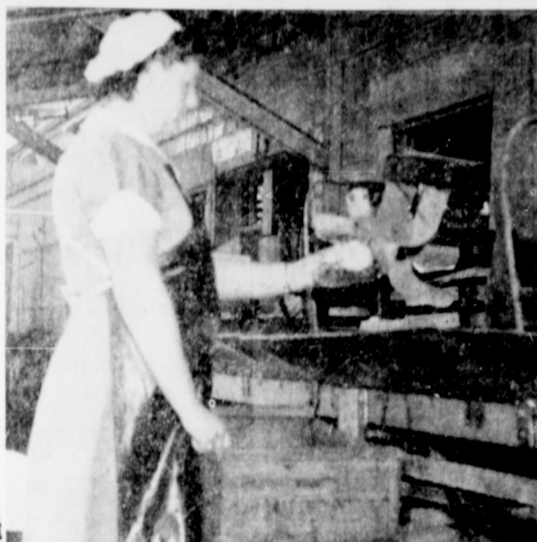
LOCAL INVENTION IN USE—Mrs. Pearl Bucher, cannery employee, demonstrates the new fruit pitting machine, recently invented by George H. Barrows of Hillsboro, whose saw-tooth blades eliminate waste and speed working time. The pitter is now in use at the B. E. Maling cannery.
