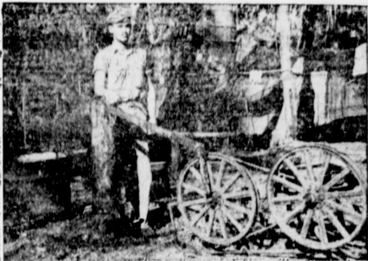
LEATHERNECK WASHING MACHINE —Laundry problems on Pacific outposts are not as difficult as one might expect. An example of Leatherneck ingenuity is demonstrated above by Cpl. Billy G. Alexander of Amarillo, Texas. The clothes are placed in the half-barrel with soap and water, and the plunger does the work. When an especially good job is desired, a fire is built under the barrel. The power? Oh, yes, propulsion is supplied by a handmade windmill.
