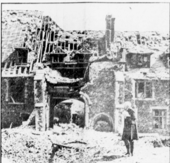
Rev. Dr. Hewlett Johnson, dean of Canterbury Cathedral, inspects damage to the Archdeacon of Maidstone's residence on cathedral grounds, after a Nazi raid.
