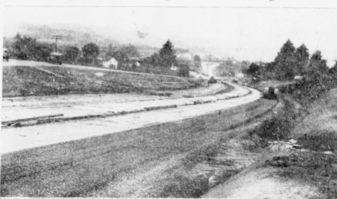
Two of four lanes on the newly rerouted 99W highway through Tigard have been poured in concrete and workmen are busy preparing the roadbed for the other half of the heavily traveled thoroughfare. The above picture, showing the stretch approaching Tigard from the east, catches two cars (in the left background) using a temporary route.—(Cut courtesy The Oregonian)
