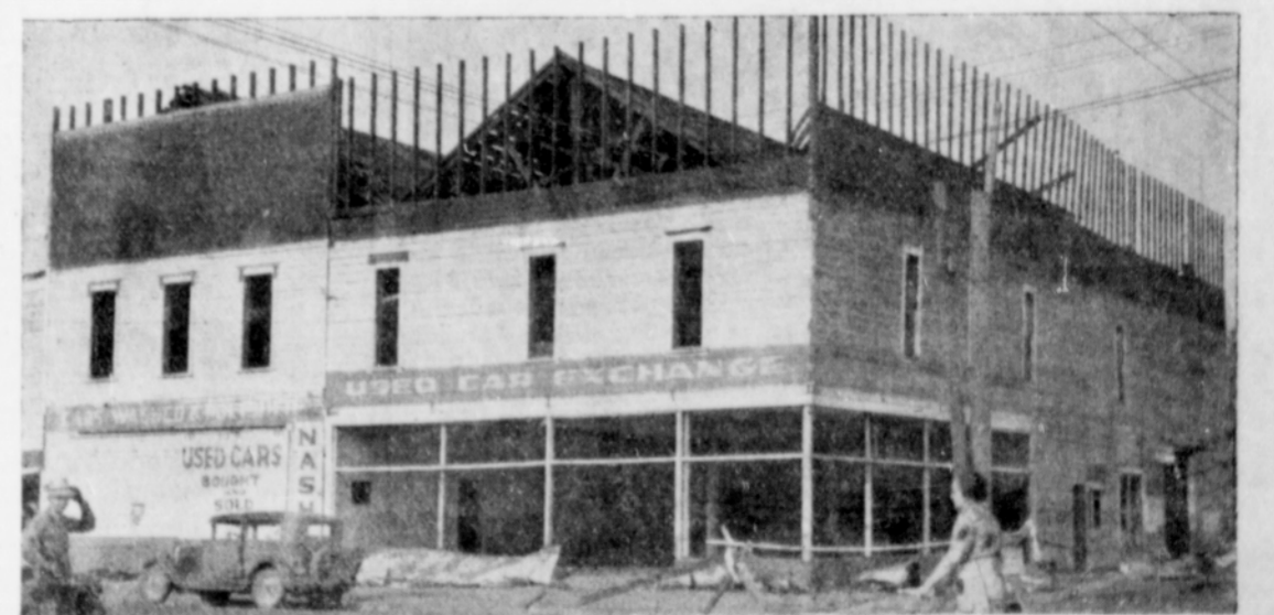
Razing of one of Hillsboro's oldest buildings got under way this week as the one-time livery barn, later a garage, on Second and Washington streets crumbled beneath the wrecker's bar to make a room for a new super-service station to be erected there. The Argus camera caught the building just after the wrecking crew had torn off the old false front which made the structure loom so large.
