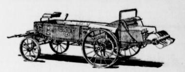
HE Case Manure Spreader is Case designed and constructed clear through. The wheels, beaters, widespreading cylinder, conveyor and other parts, are all built by Case into a complete and efficient spreader.
