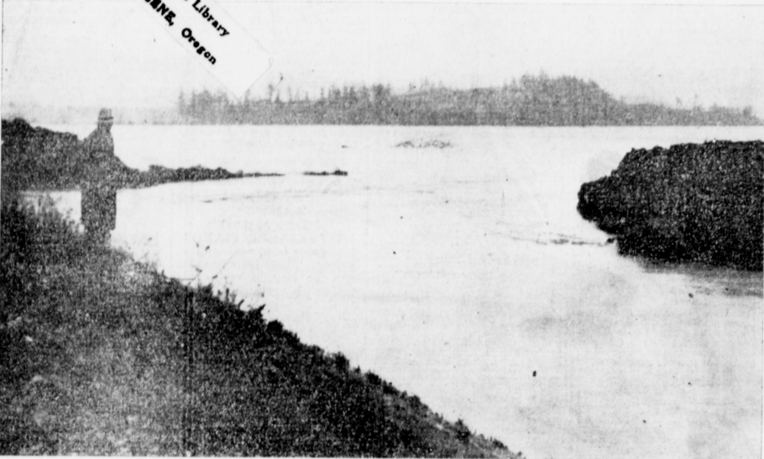
Flood waters covered Wapato lake as of old Tuesday night after raging floods had torn a 60-foot hole through the $75,000 dike, intended to keep the lake bed dry. Gaston in the foreground is the swollen moat outside the dike and the break in the wall. Flooded area in the background was an onion field a few days ago. This also eased the flood condition further along the Tualatin river valley. Cut courtesy Oregonian.
